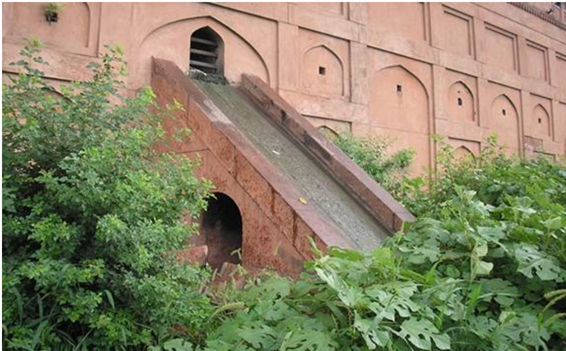
Figure 11. A view of rainfall passage of rainfall exist from Badshahi Masjid Lahore.
