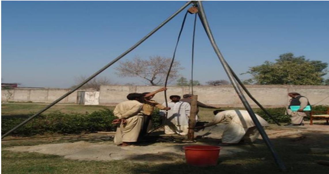
Figure 6. Drilling of exploratory boreholes in field.
